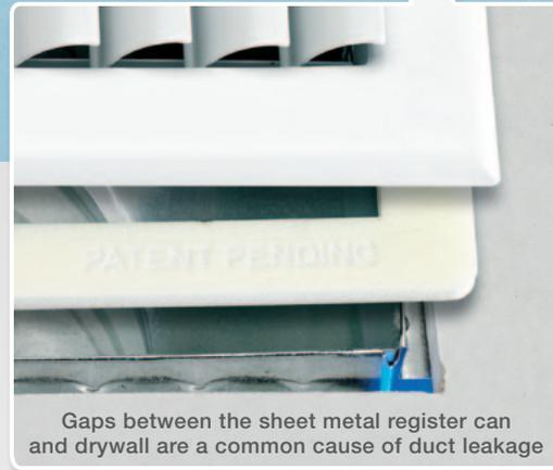
Gaps between the sheet metal register can and drywall are a common cause of duct leakage
